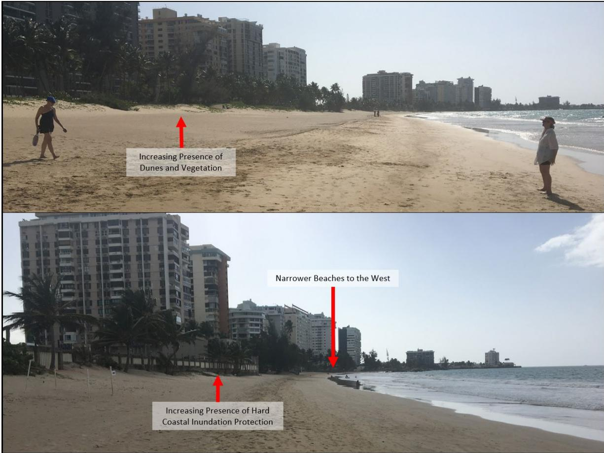
**Figure A - 15. Decreasing Beach Widths and Increasing Flood Protection near IV6/IV7, Facing West**
