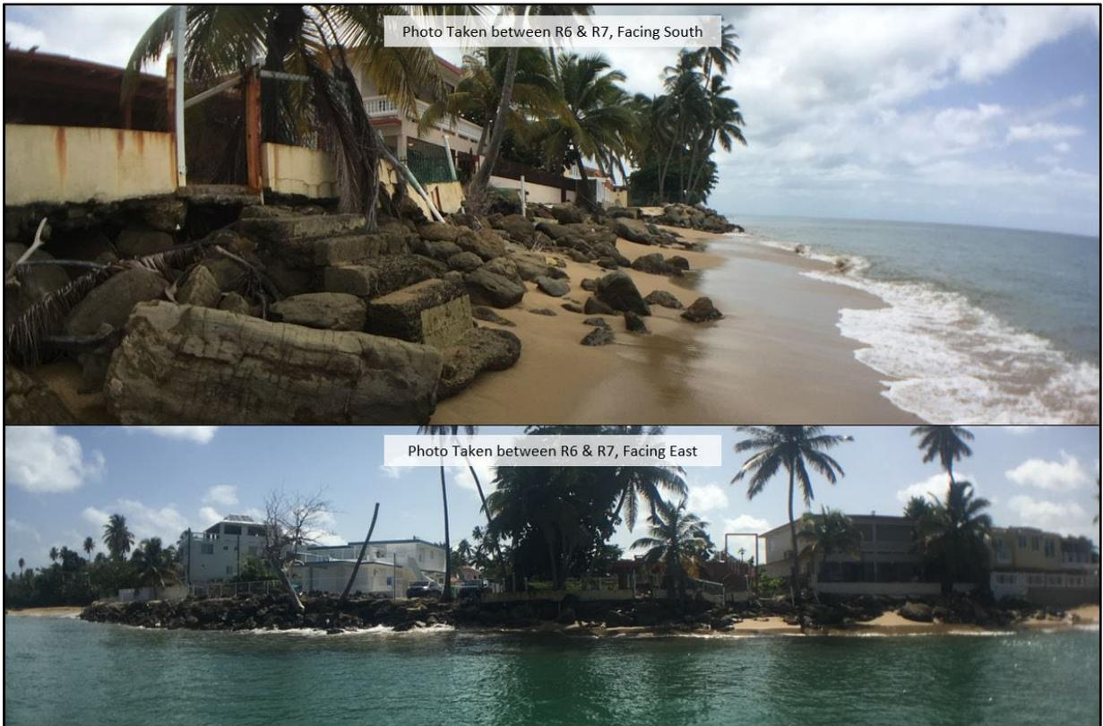
**Figure A - 38. Rock Revetment and Debris in front of Small Seawalls near R6/R7**
