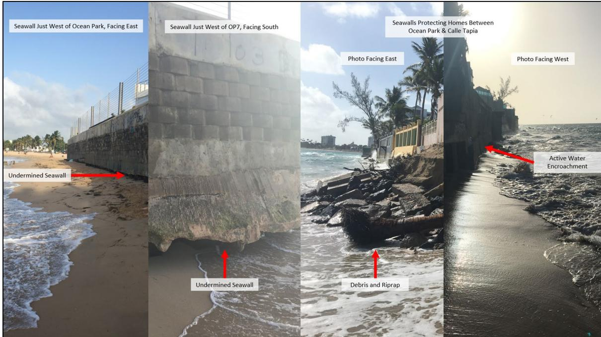
Figure A - 22. Ocean Water Encroachment and Undermined Seawalls Just West of Ocean Park
