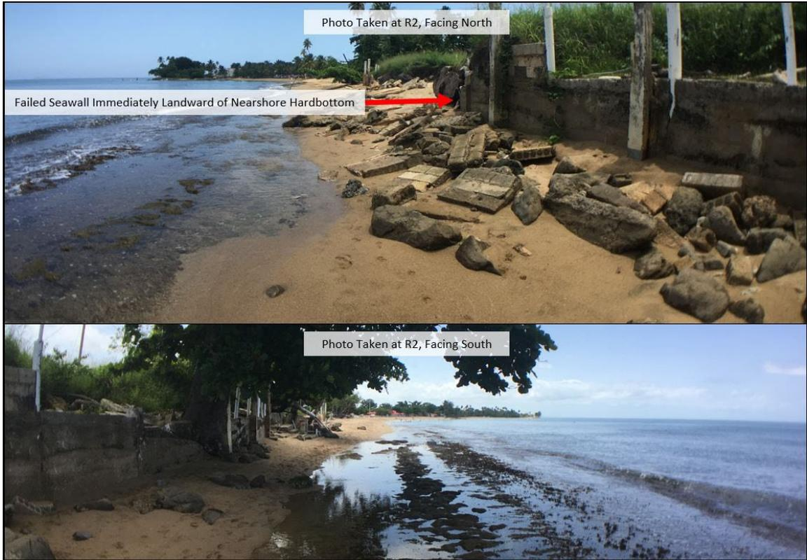
**Figure A - 34. Failed Seawall and Nearshore Hardbottom near R2**
