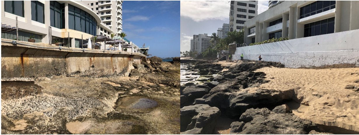
Pictures from left to right: Robust seawall tied into the bedrock in Planning Reach Condado West Headland; Robust emergent seawall with buried foundation in Condado Punta Piedrita
