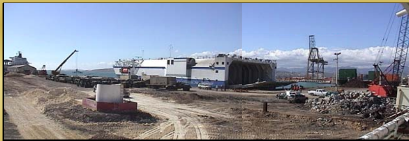
Improvements to Piers 4, 5, 6 & 7 at Port of Ponce
