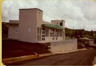
Improvements to Agricultural Infrastructure in Orocovis
