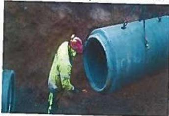
Water Drain System (Concrete Pipes)
