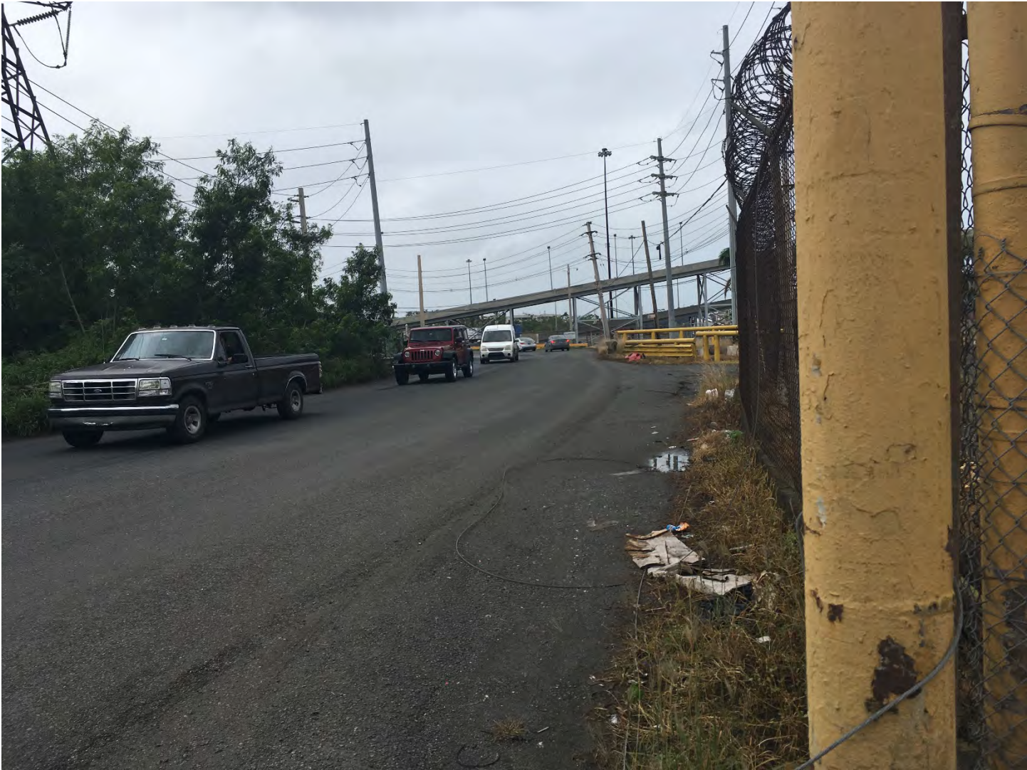
Fence and Brush partially obstruct view for exiting vehicles. Available Sight Distance limited to approximately 250 Feet.
