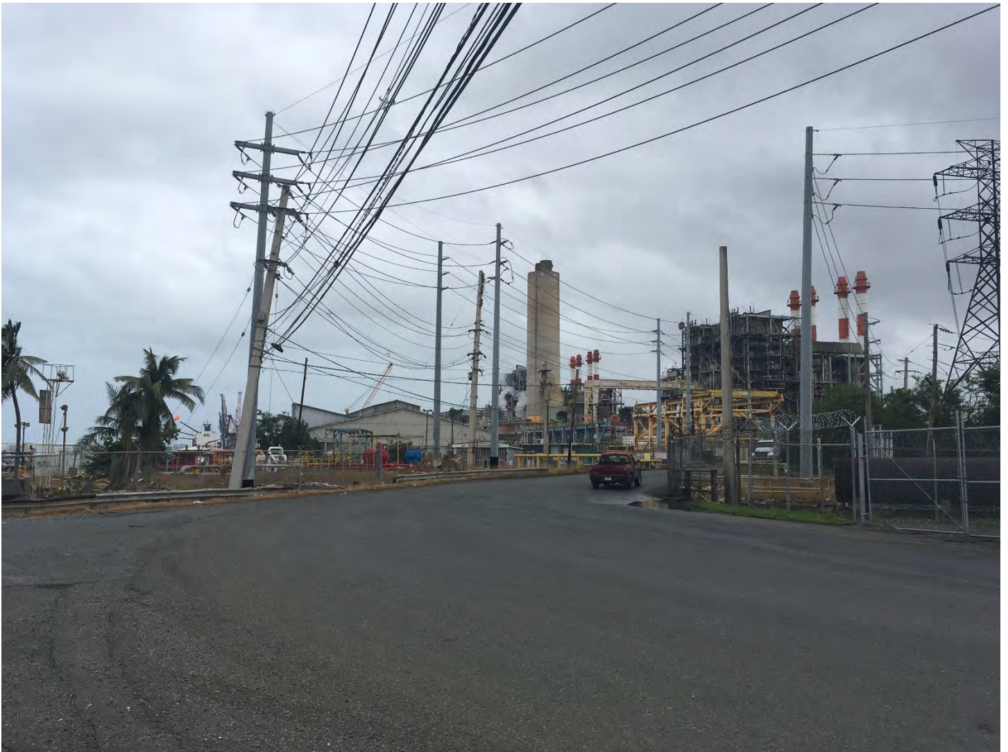
Sharp Corner on Route 28 just before access driveway to Wharves A & B (can't see driveway or vehicles waiting to turn left into Access driveway to Wharves A & B)
