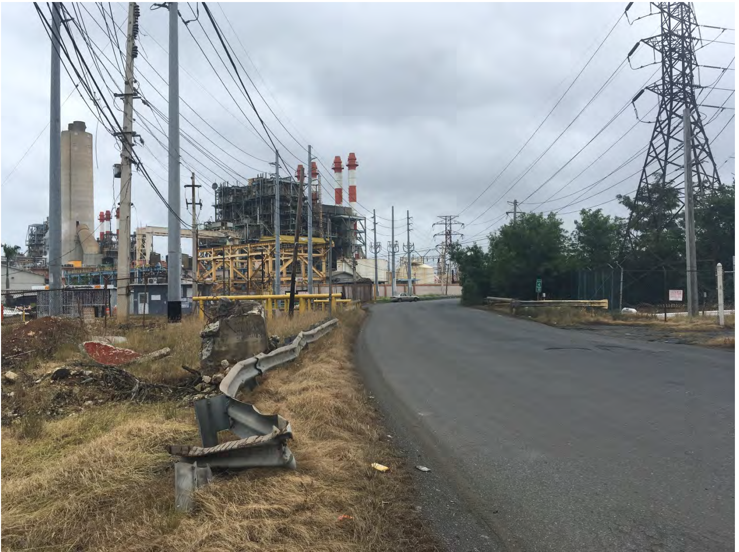
View facing Access driveway to Wharves A & B from Route 28 (can't see driveway or vehicles waiting to turn left into Access driveway to Wharves A & B)
