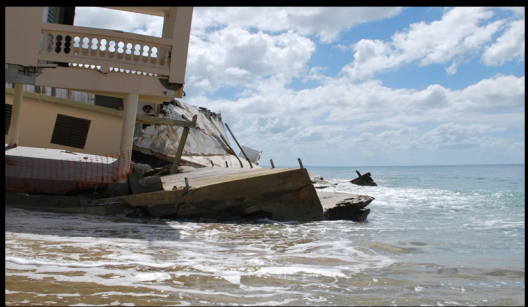
Severe erosion & wave attack, Rincon
