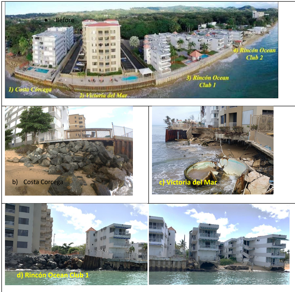
Figure 2-17. Severe damage to properties generated by Hurricane Maria in Rincón
